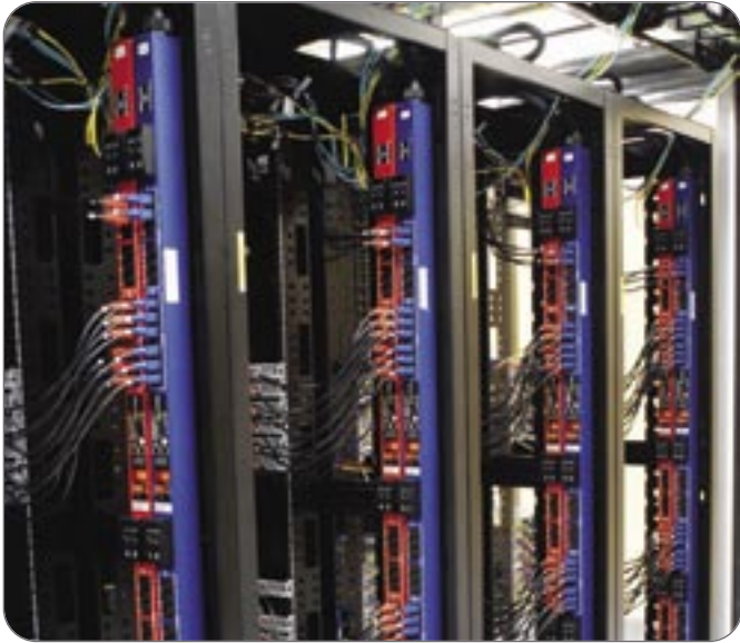
Raritan's Dominion PX family of rack PDUs provides accurate, real-time kilowatt-hour information for each individual asset in the data center.
